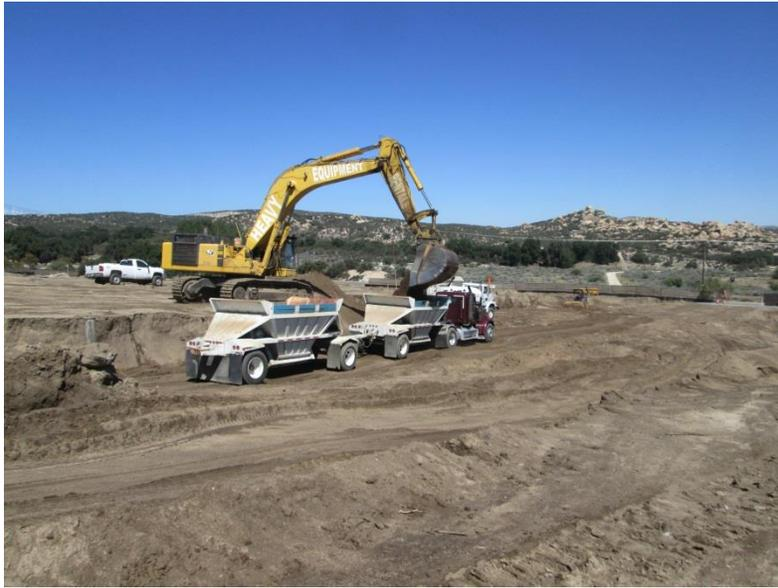
**Photo 3:** An excavator is utilized to load haul trucks to export soil from the Boulevard Substation Rebuild Site.
