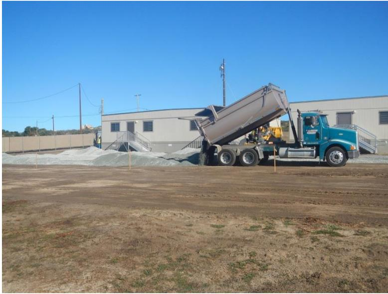
**Photo 5:** Gravel base being delivered to the Jewel Valley Construction Yard that will be utilized to stage construction equipment and materials.
