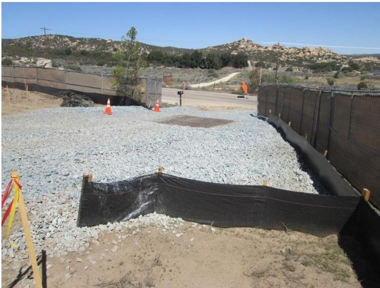
**Photo 4:** Trac-out measures consisting of a rattle plate and rock apron are being maintained at the point of ingress/egress to the Boulevard Substation Rebuild Site along Old Highway 80.
