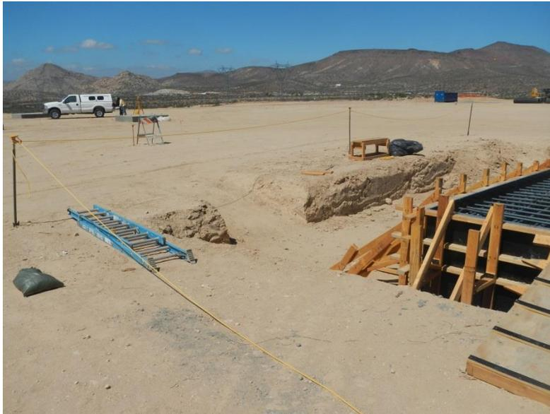
**Photo 2:** Wildlife escape ramps being utilized at the 138/230 kV ECO Substation pad site to prevent wildlife entrapment in accordance with MM-BIO-7A.
