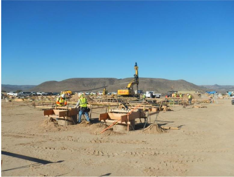
**Photo 1:** Construction crews completing concrete foundations for substation components at the 138/230 kV ECO Substation pad.
